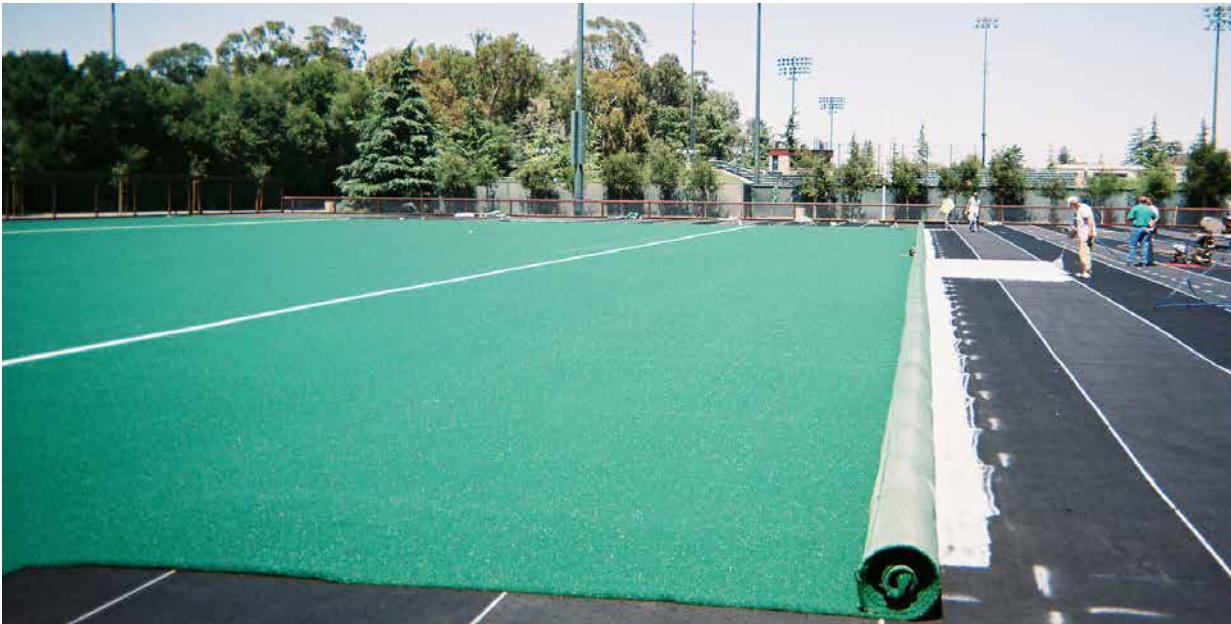
Stanford University installation in progress
