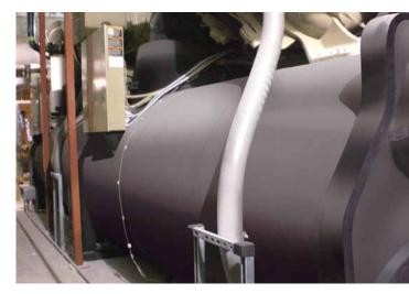
It is structurally resistant to tears and it will not absorb moisture, which means that it doesn't require any type of vapor barrier.
