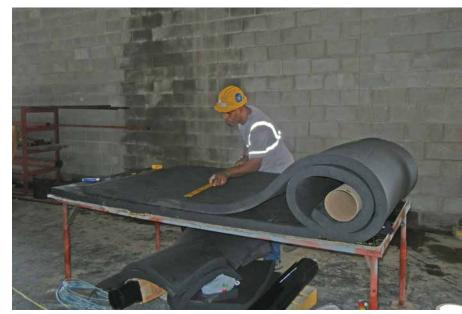
With this ready crew of skilled labor, Integ was able to set up an efficient pre-fabrication station within Integ's temporary warehouse located at airport jobsite. In this controlled environment, workers were able to pre-insulate all the piping (3/4 to 16-inch) and pre-fabricate Armaflex fitting covers using templates provided by Armacell.
