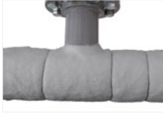
Figure 46: Insulate main pipe around branch.
