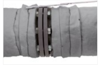
Figure 31: Wrap 50 mm (2 in.) wide strips of ArmaGel HT to build up insulation to clear flange (or adjust width to be equal to total insulation thickness if > 50 mm).
