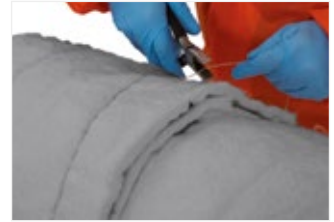
Figure 33: Wire in place.
