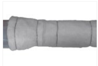
Figure 45: Butt pipe insulation tightly up to reducer.
