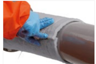
Figure 12: Longitudinal overlapped seam.
