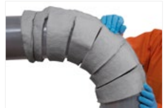
Figure 39: Position cut outs on inside throat of bend with longitudinal joint on outside of bend.
