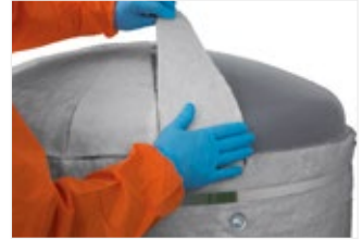
Figure 61: Apply closely-butted segments and fix using insulation stick pins and bands.
