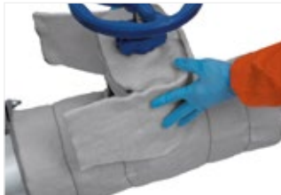
Figure 58: Wrap valve stem.
