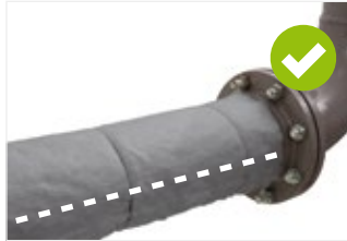
Figure 17: Rotate longitudinal seam to side.
