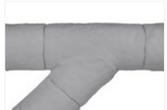
Figure 53: Install oblique angled branch and wire into place ensuring that all joints are tight without gaps.
