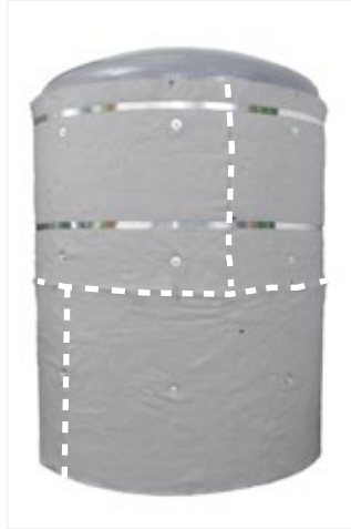
Figure 60: Insulate from the vessel head weld line. Hold ArmaGel HT sheet with insulation stick pins, staggering all joints, then band each layer to vessel.
