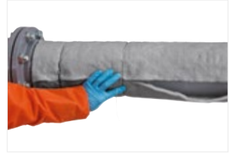
Figure 14: Continue to make seam, closing gaps.
