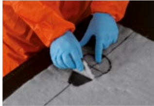
Figure 50: Create cut out for oblique angled branch.
