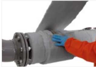
Figure 32: Wrap to same thickness as ArmaGel HT on pipe.
