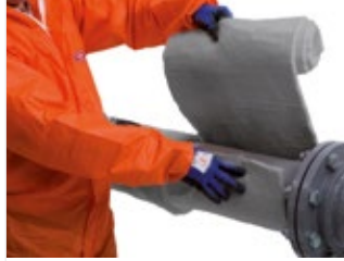
Figure 24: Ensure starting point is in line with axis of pipe. Tape or adhesive may be required to help hold the axial position.
