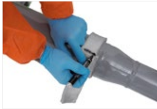
Figure 42: Measure both circumferences over the weld.
