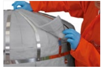
Figure 62: Joints in subsequent layers should be staggered.
