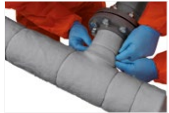
Figure 49: Wire into place.
