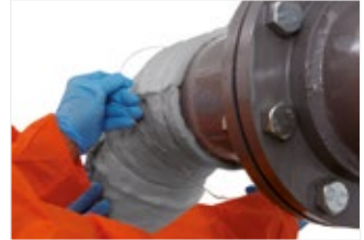
Figure 35: Ensure all joints are closely butted without gaps and that they fit the pipe tightly without voids.
