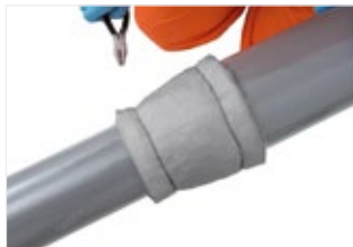
Figure 44: Fit around reducer and wire in place.
