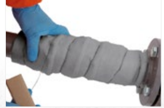
Figure 29: Spiral wrap with wire to hold ArmaGel HT in place.
