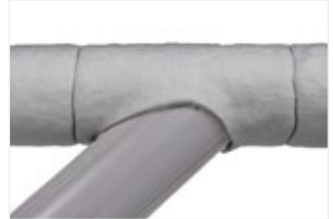
Figure 51: Wrap around pipe and wire in place.
