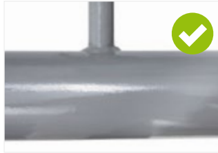
Figure 7: Ensure that piping is clean, dry and free from ice.
