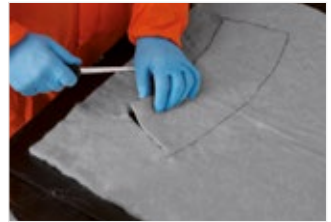
Figure 43: Cut radiused strip.
