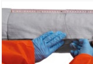
Figure 15: Secure with wire.
