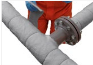
Figure 48: Install branch piece.
