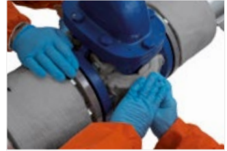
Figure 55: Pack ArmaGel HT around body of valve to prevent voids.
