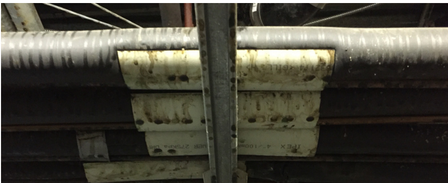
1 Example of a shifted saddle as well as saddles that are too small
