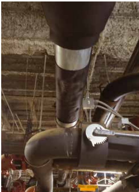
Insulation cell collapse due to CUI on pipes masked by the insulation.
